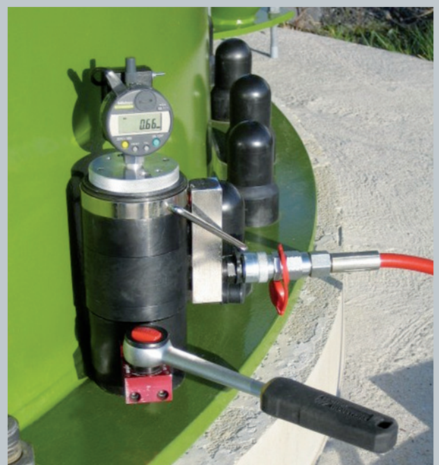
Picture 8: Tensioning of Foundation bolts
